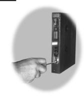
Insert lockbody (and hookbolts for Triad) into door prep. Check that lock fits easily in door with screw holes aligned.
