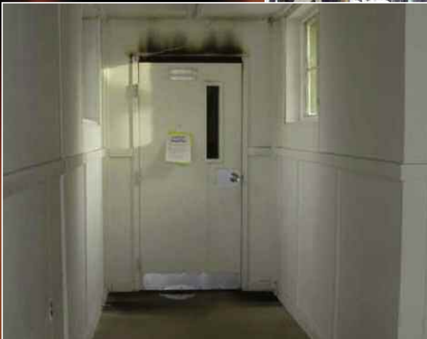
The Same Fire Door kept this section of the building safe
