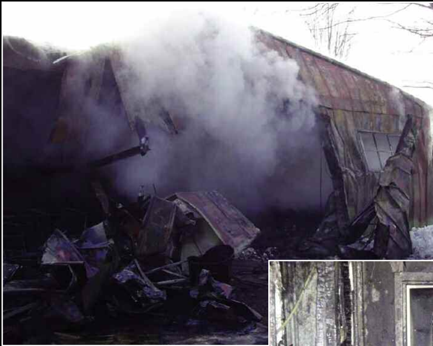
Damage sustained to a portion of the building
