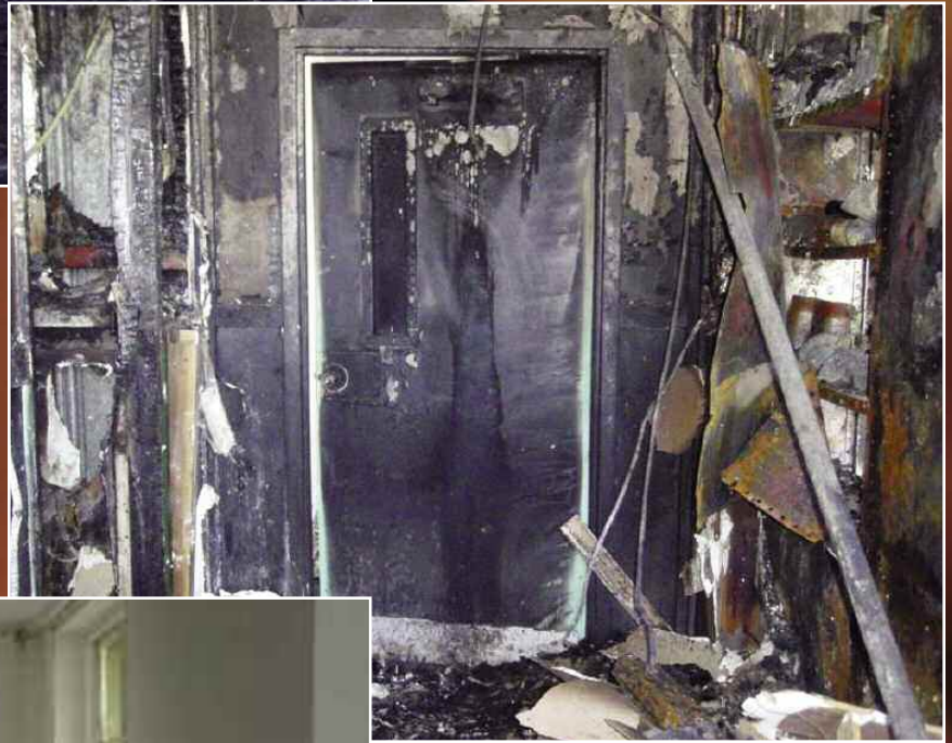
Fire Door Where Fire Originated
